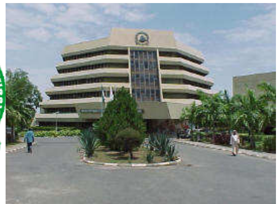
NUC Headquarters in Abuja
